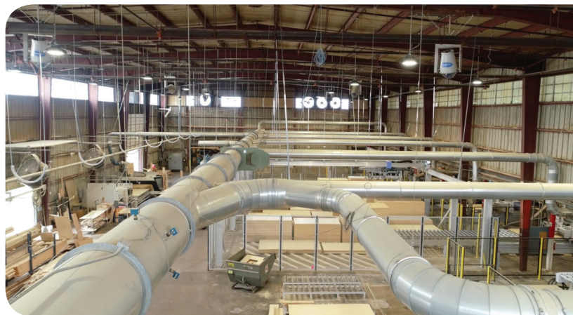
After installation and use of a SonicAire dust control system to clear away combustible dust.
