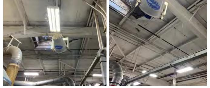
Columbia Forest Products uses a system of 10 SonicAire fans to keep their plant ceiling and rafters clean and displace dust to the floor, where they are able to sweep the dust up and take care of it on a daily basis.
